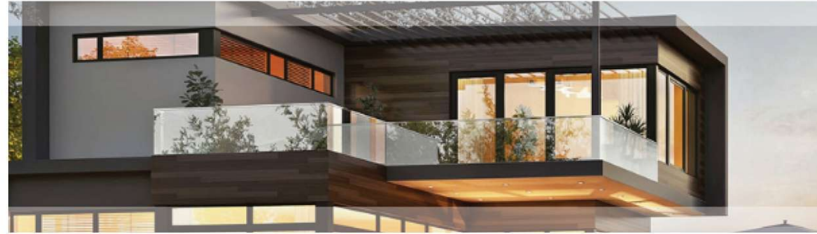
Other System- Handrail
